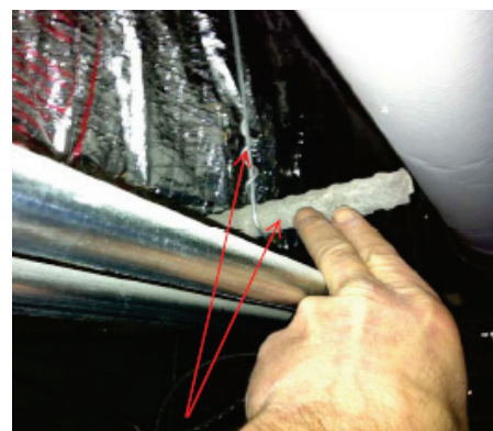
Figure 32 – Rebar & Wire Used for Duct Support
