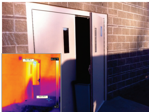
Figure 12 – Propped Open Rear Entry Door
