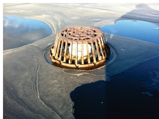
Figure 10 – Scupper Drain (note drain pipe invert is 2" above deck)
